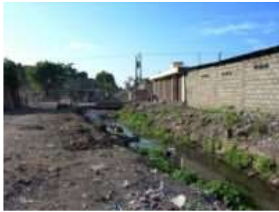
Outpourings of sewage like this...
